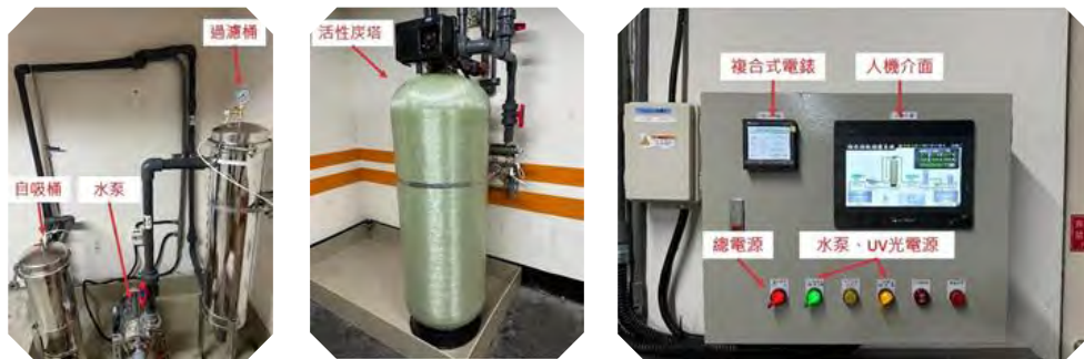
▲ Rainwater Harvesting System Equipment Configuration Diagram
